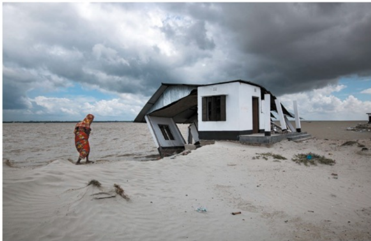
A damaged temporary home near the Meghna River in Bangladesh, in a coastal area threatened by erosion and rising saltwater levels in soil.
