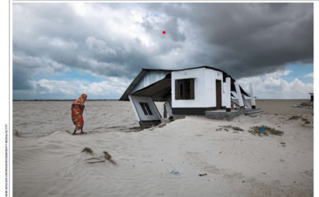
A damaged temporary home near the Meghna River in Bangladesh, in a coastal area threatened by erosion and rising saltwater levels in soil.
